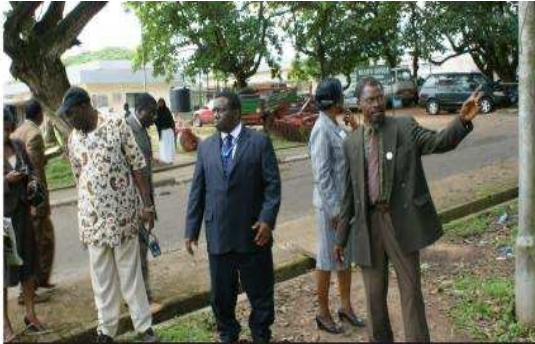
Dean of Agric & Forestry, Prof. E. A. Aiyelari showing damaged structures to the VC & his Team
