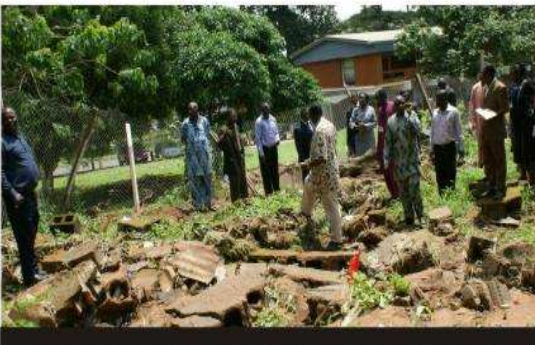
Damaged fence behind the Department of Forest Resources Management
