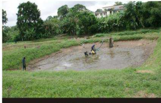
Washed away Fish Pond
